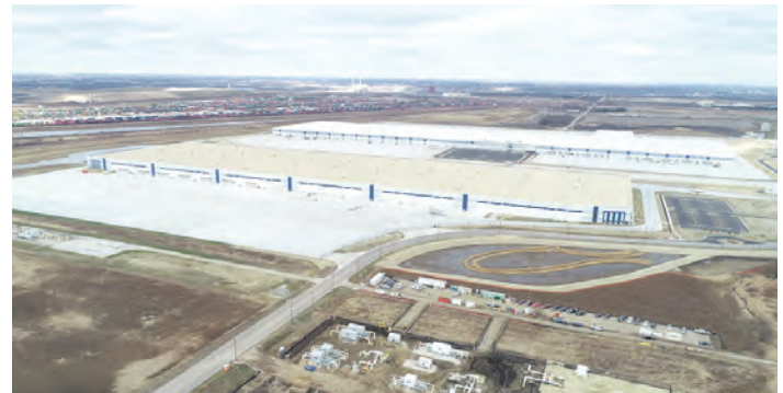
3501 NORTH BRANDON RD., CENTERPOINT INTERMODAL CENTER-JOLIET, IL
